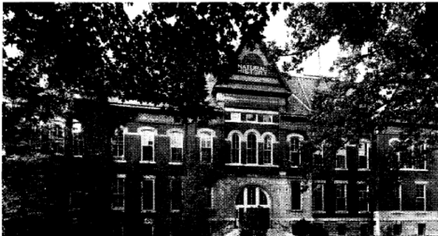
Figure 1. The Natural History building from the north. Physiology occupied part of the fourth floor from 1892 to 1959.
