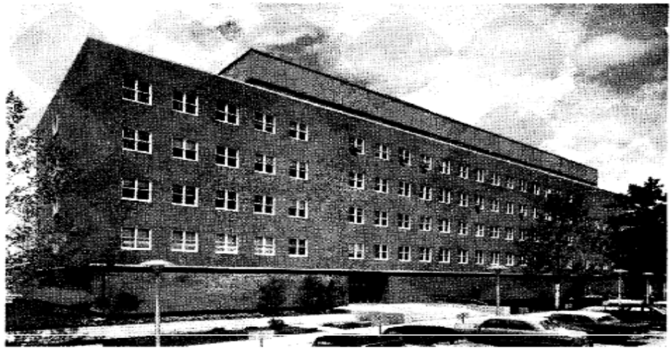
Figure 2. Burrill Hall from the southwest. Physiology moved into the fourth and fifth floors and half of the basement in 1959.
